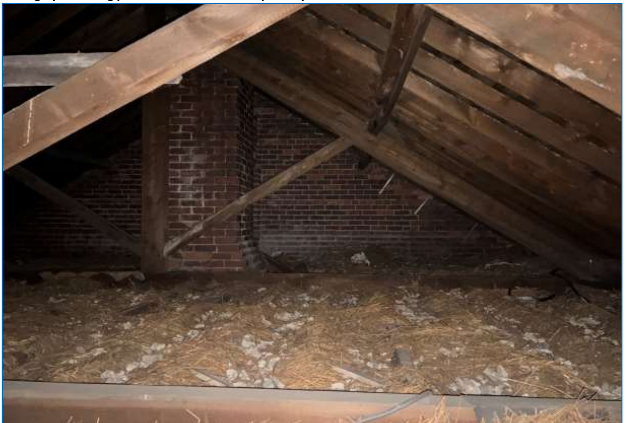
Photograph 6 – King post roof void with straw possibly used for insulation.
