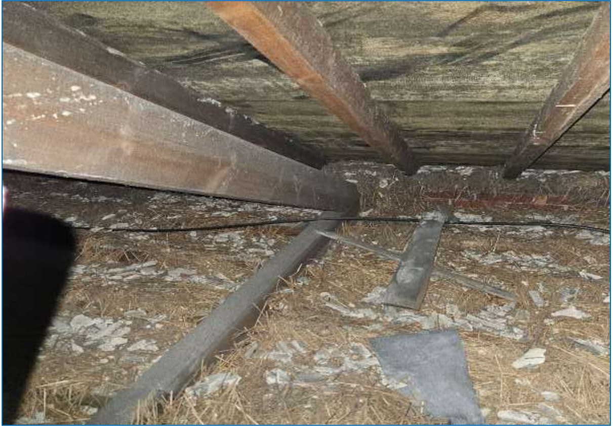
Photograph 7 – The main building roof void was generally cool and dusty.
